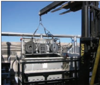
Figure 3. First set of dies removed from the cleaning tank. (At this point in time forklift was being used because overhead crane had not yet been installed.)
